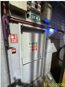
FU-ONE OF EMERGENCY EXIT DOOR.JPG
